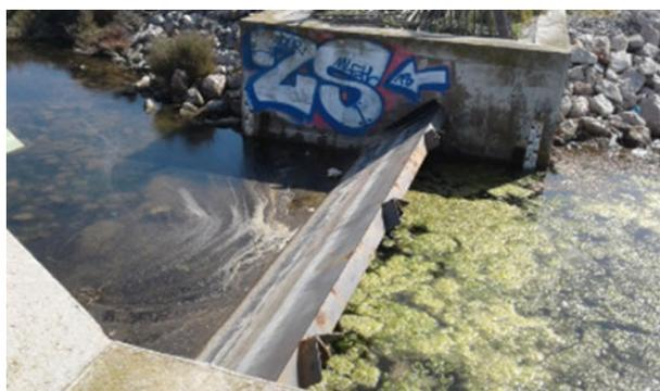
Photo d'un clapet basculant – Mathilde AMAND, AFB
